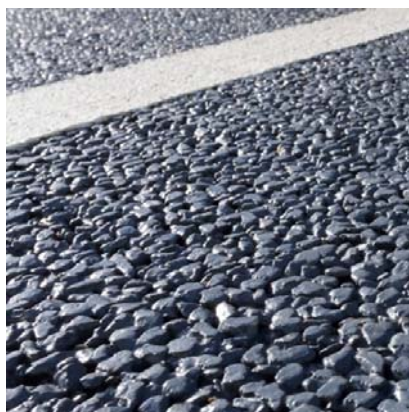
Macadam; preferably permeable to assist with sustainable drainage (image copyright Tarmac)
