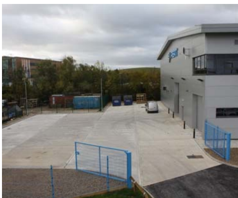
Concrete to service yards only (image copyright M&H Groundworks)
