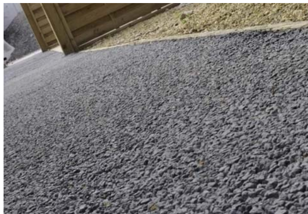
To footpaths away from building frontages: Macadam; preferably permeable to assist with sustainable drainage (image copyright Tarmac)
